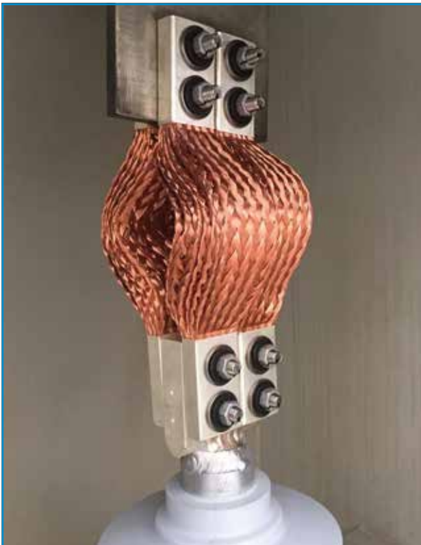
Copper braids to transformer
