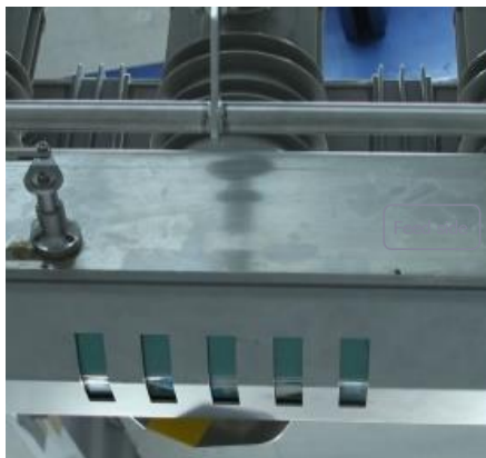
Bottom switch position indicator
